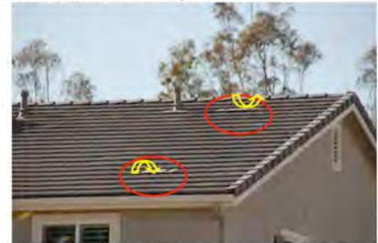
Eave vents are eliminated and moved to the roof. Vent location is in the lower portion of the roof – other venting must be installed close to the ridge (or ridge vents used).
